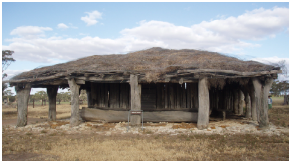
Clayton Farm thatch shed, red gum posts and trough
